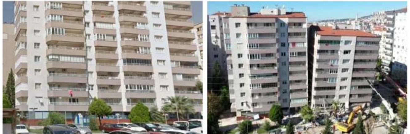
Fig.2: Damages in Izmir
