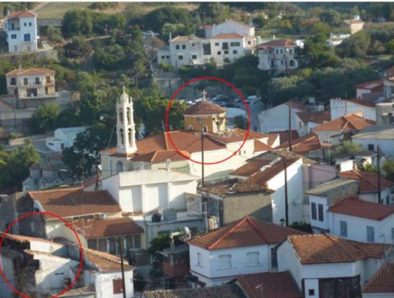
Fig. 1: Damages in Vathy
